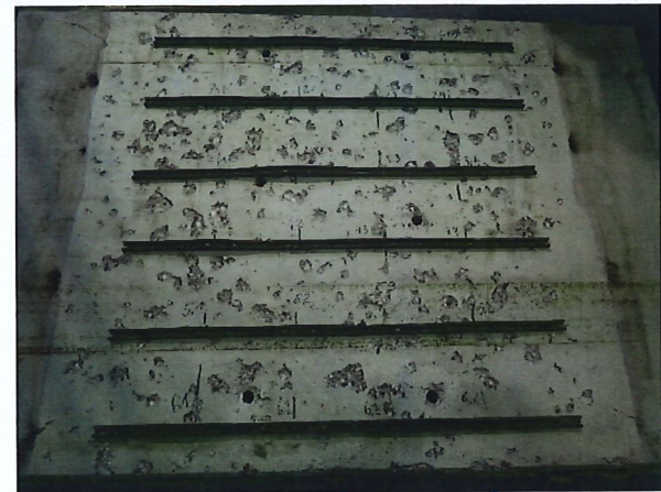
Figure A4.9 View of the installation bars after the fire test.
